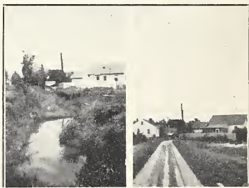
FIG. 4. Grenada, Mississippi. Left, before malarial control drainage; right, after construction of brick and mortar invert with sodded banks.
